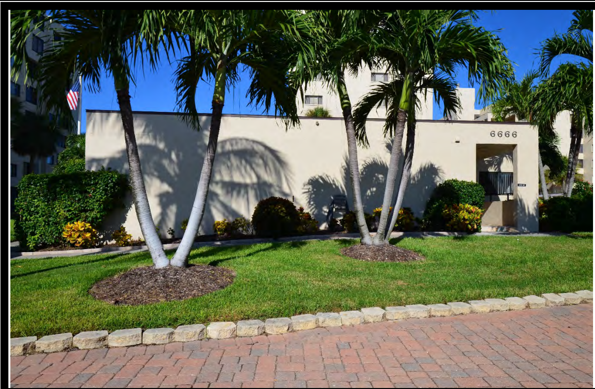
VIEW OF OFFICE/MANAGER'S APARTMENT
