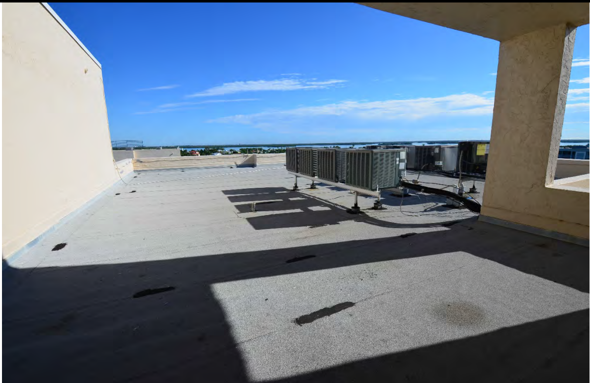
VIEW OF TYPICAL ROOFS
