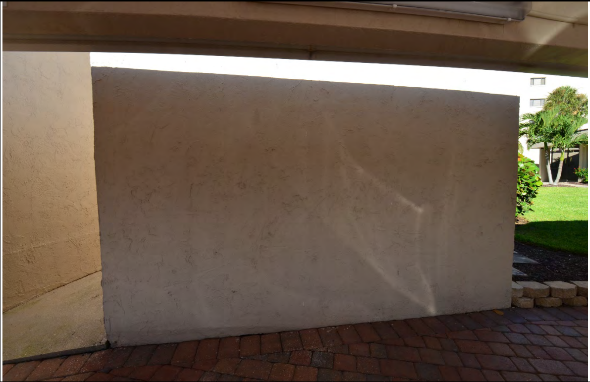
VIEW OF GENERATOR BUILDING
