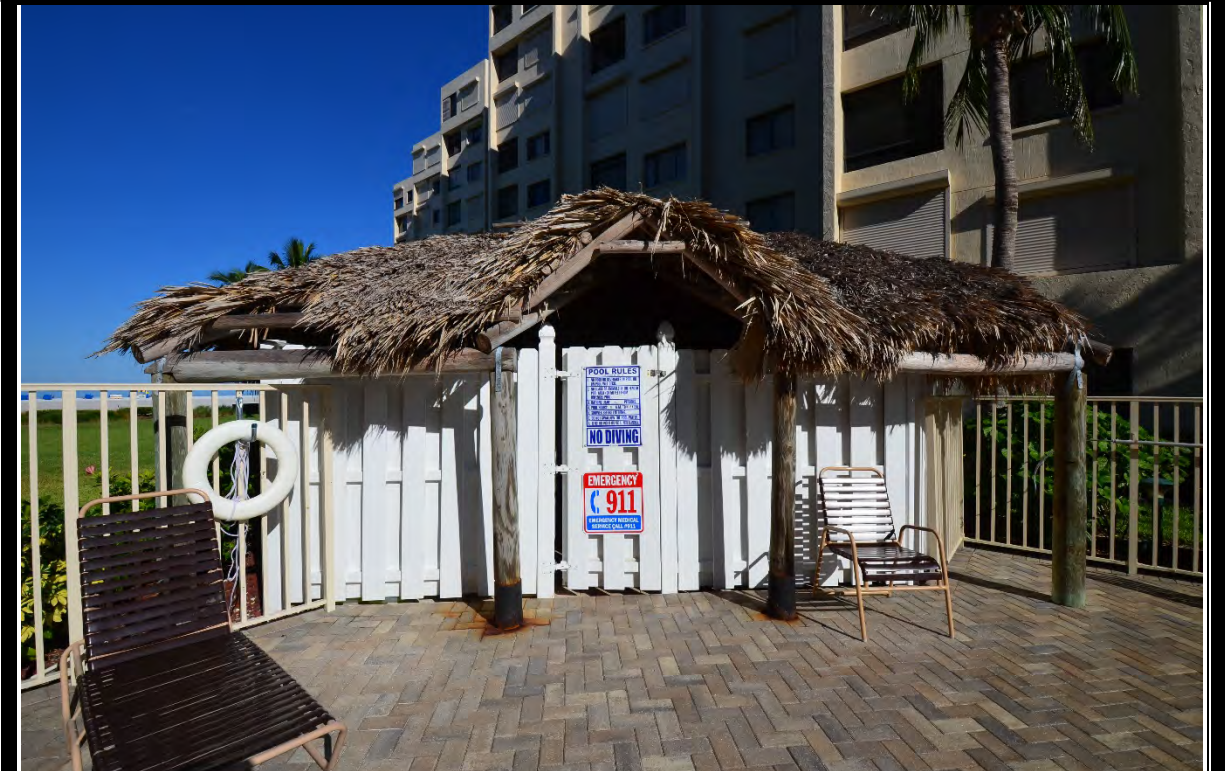
VIEW OF POOL EQUIPMENT CABANA
