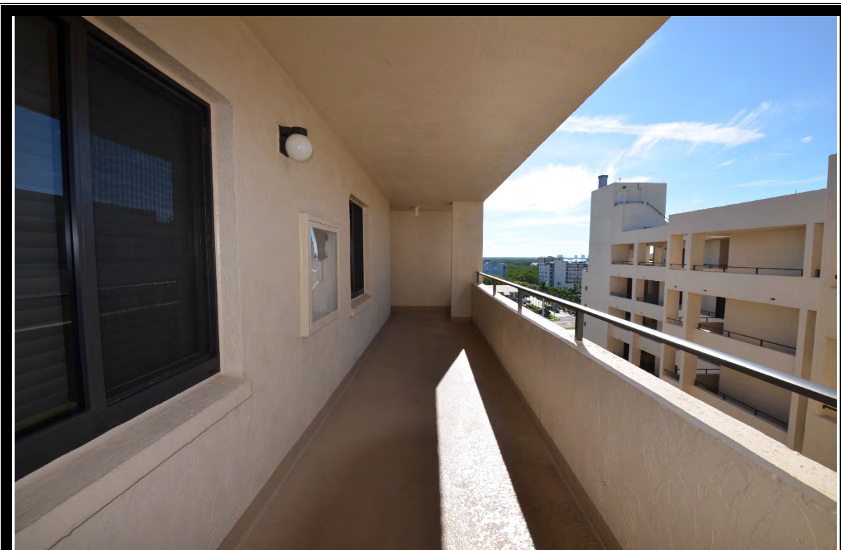
VIEW OF TYPICAL COMMON AREAS
