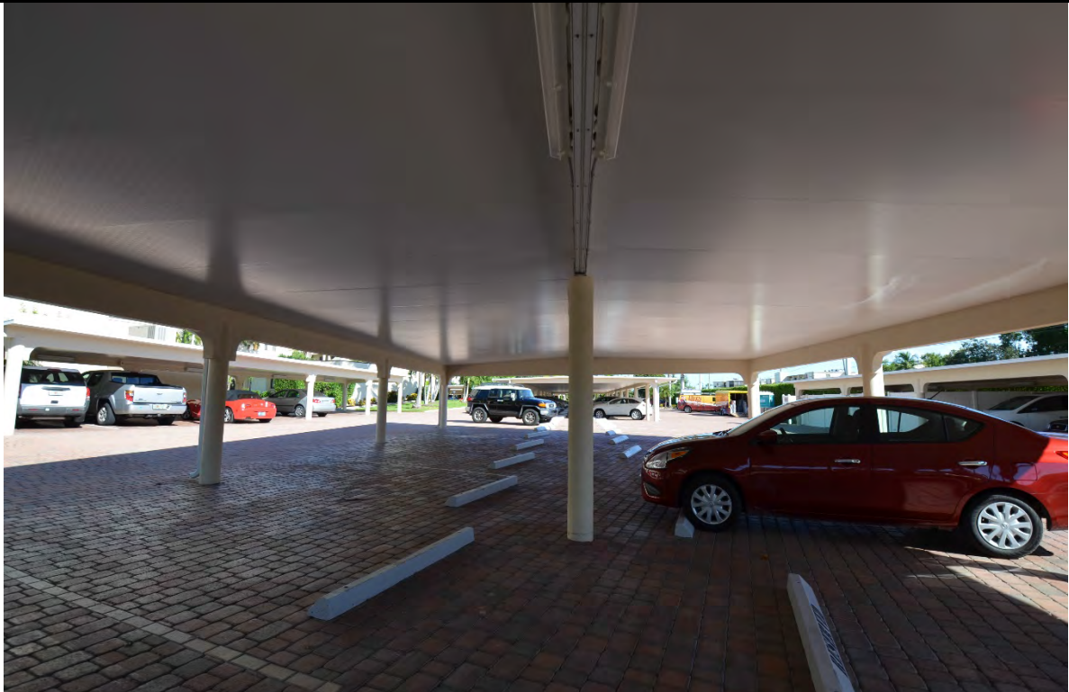
VIEW OF TYPICAL CARPORT STRUCTURES
