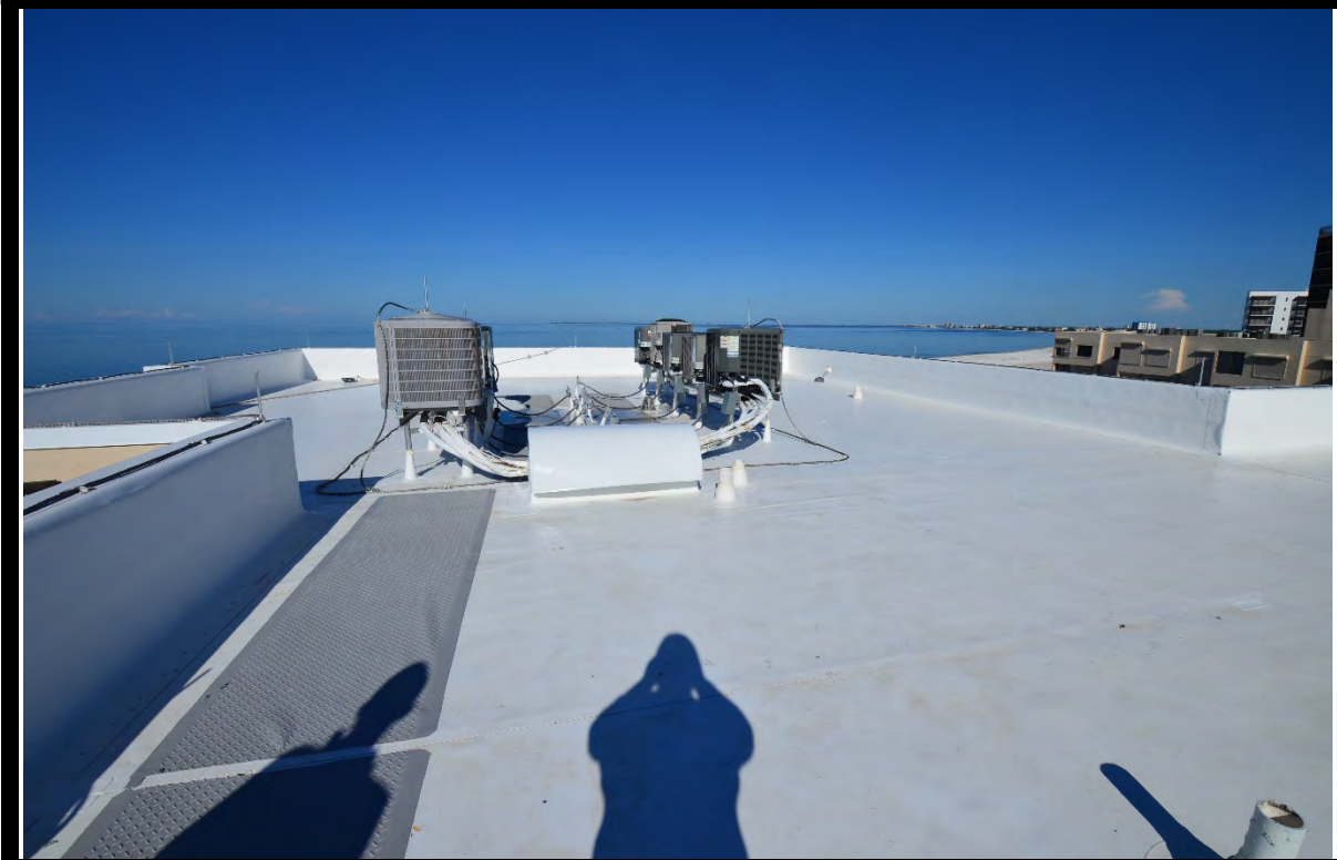
VIEW OF TYPICAL ROOFS
