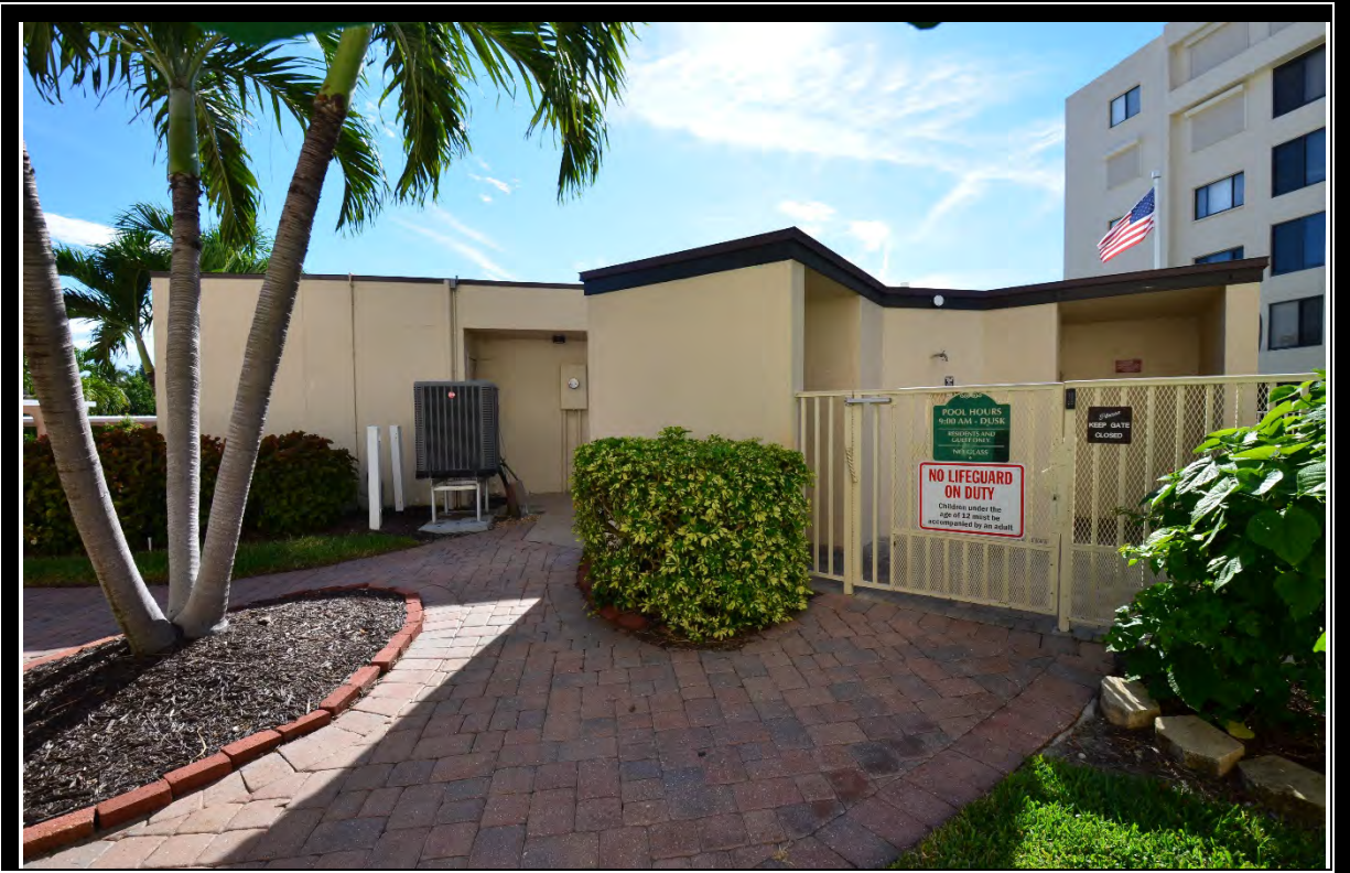
VIEW OF OFFICE/MANAGER'S APARTMENT
