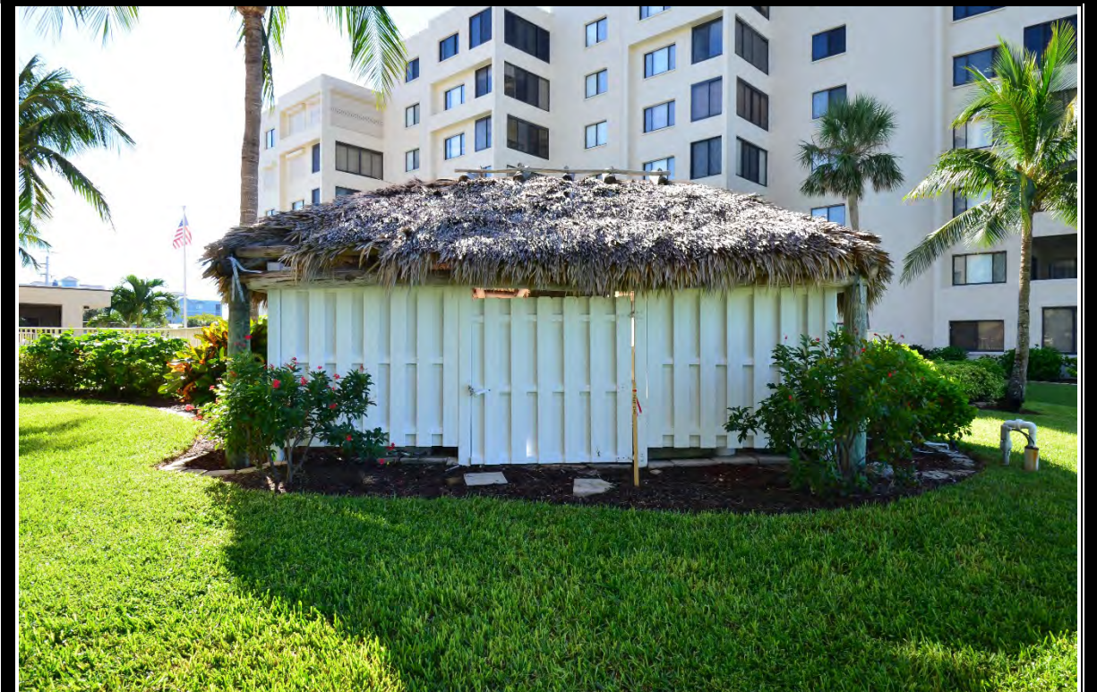
VIEW OF POOL EQUIPMENT CABANA
