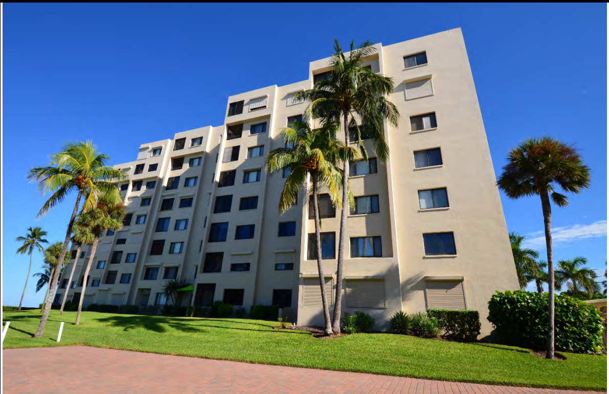
EXTERIOR VIEW OF 6672 ESTERO BOULEVARD 50 UNIT RESIDENTIAL BUILDING
