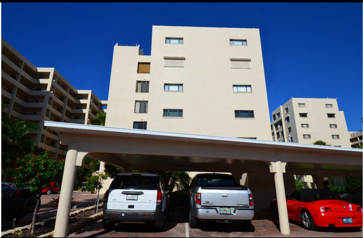
EXTERIOR VIEW OF 6670 ESTERO BOULEVARD 38 UNIT RESIDENTIAL BUILDING
