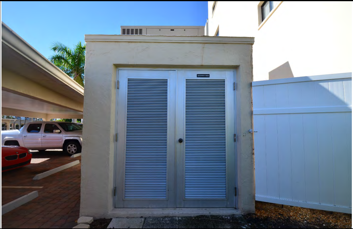
VIEW OF GENERATOR BUILDING
