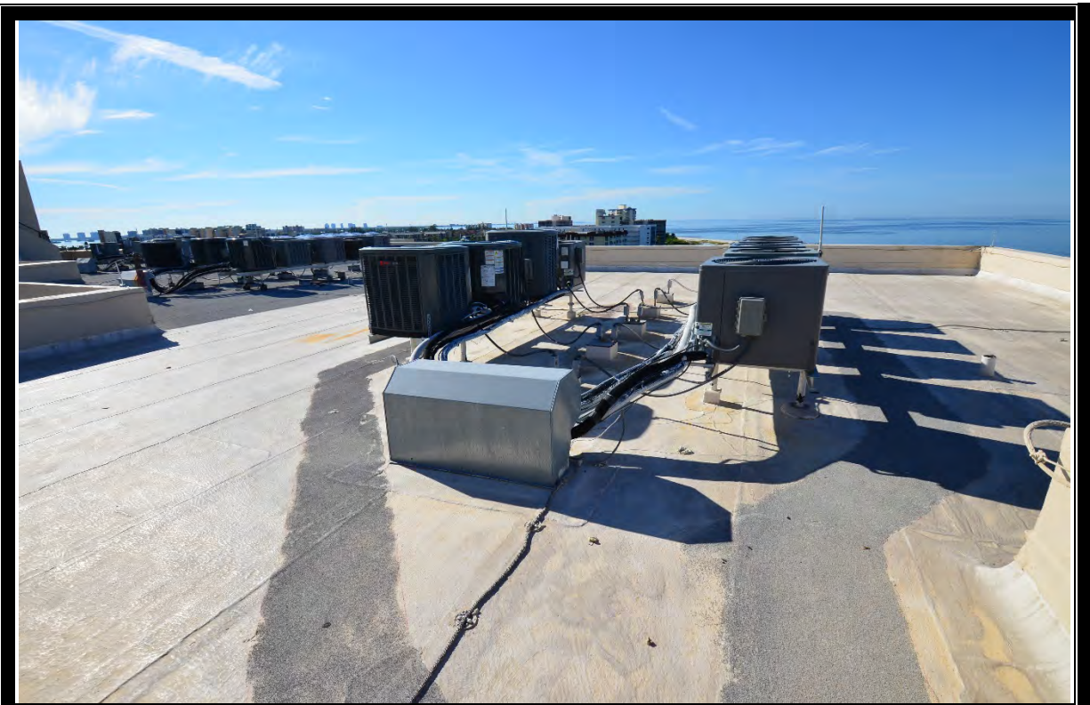
VIEW OF TYPICAL ROOFS
