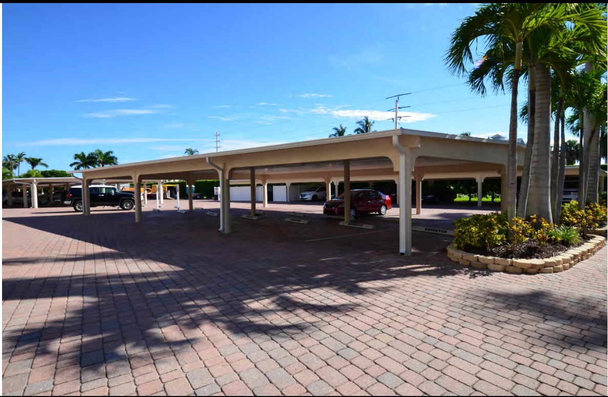
VIEW OF TYPICAL CARPORT STRUCTURES
