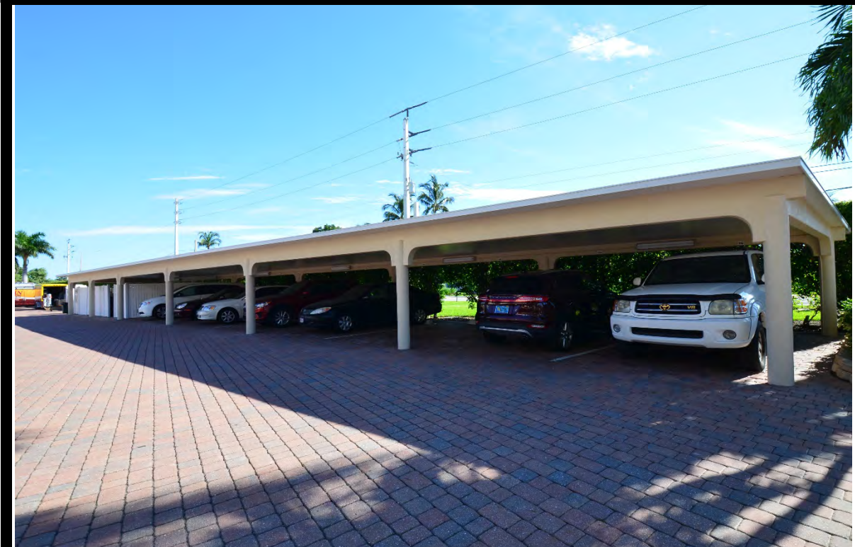
VIEW OF TYPICAL CARPORT STRUCTURES
