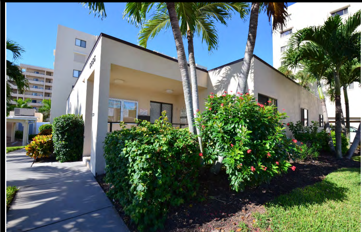
VIEW OF OFFICE/MANAGER'S APARTMENT
