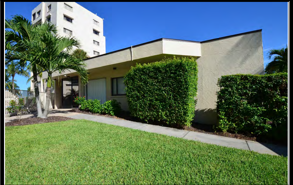
VIEW OF OFFICE/MANAGER'S APARTMENT
