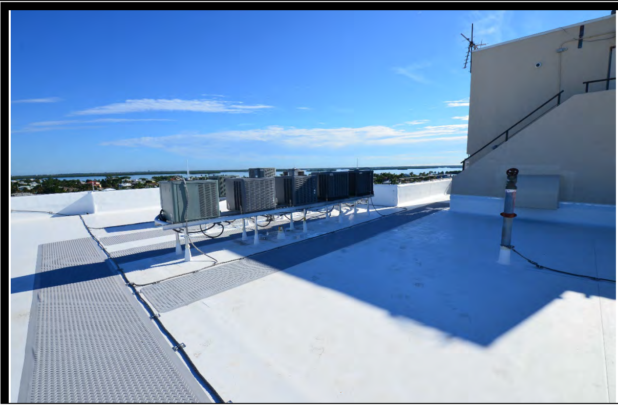
VIEW OF TYPICAL ROOFS
