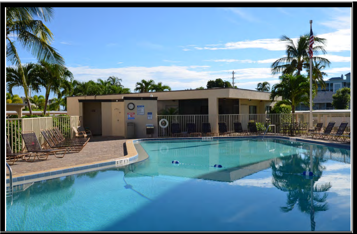
VIEW OF OFFICE/MANAGER'S APARTMENT
