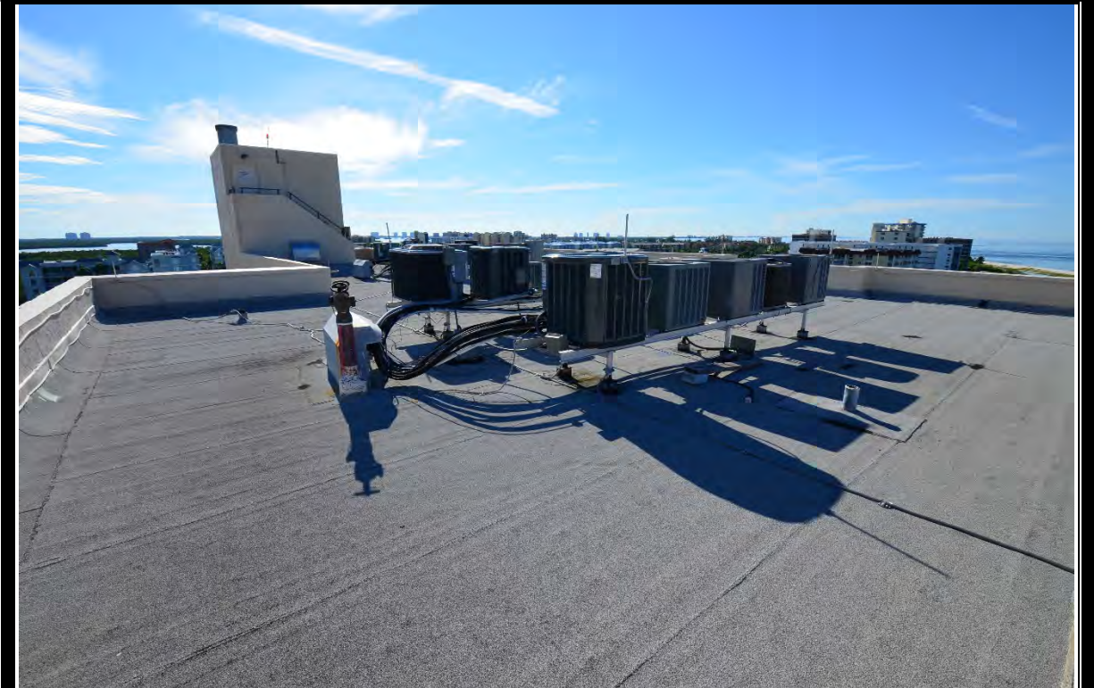
VIEW OF TYPICAL ROOFS
