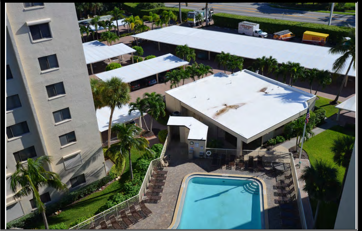
VIEW OF OFFICE/MANAGER'S APARTMENT
