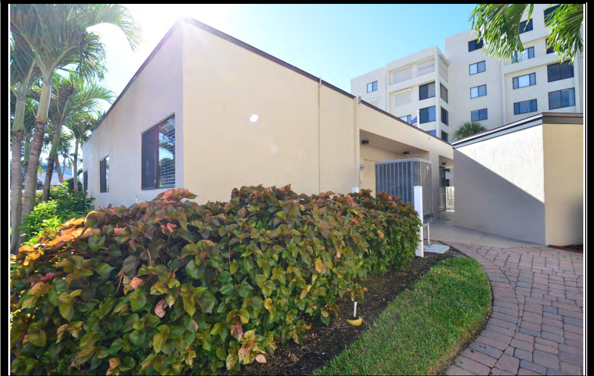
VIEW OF OFFICE/MANAGER'S APARTMENT
