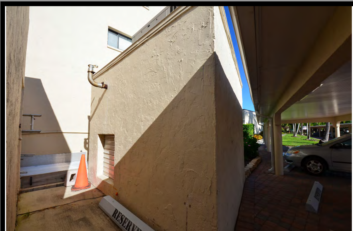
VIEW OF GENERATOR BUILDING
