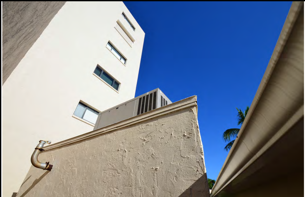
VIEW OF GENERATOR BUILDING
