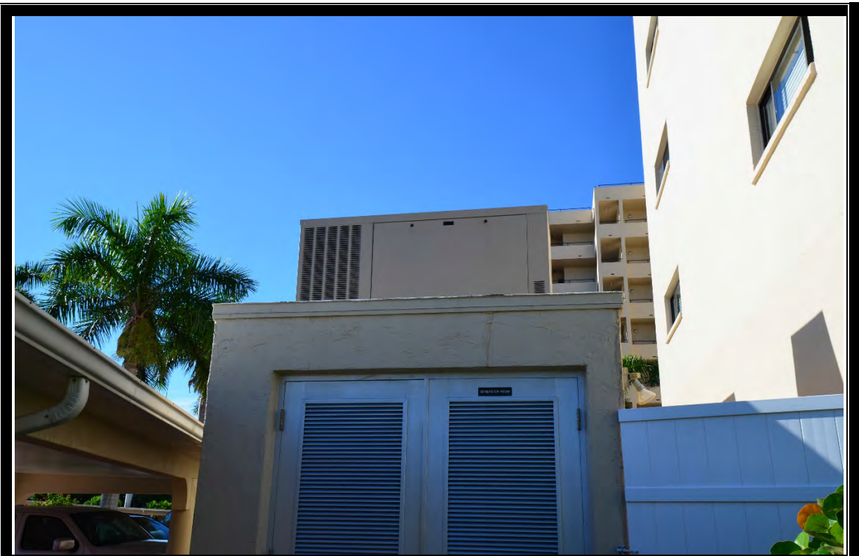
VIEW OF GENERATOR BUILDING
