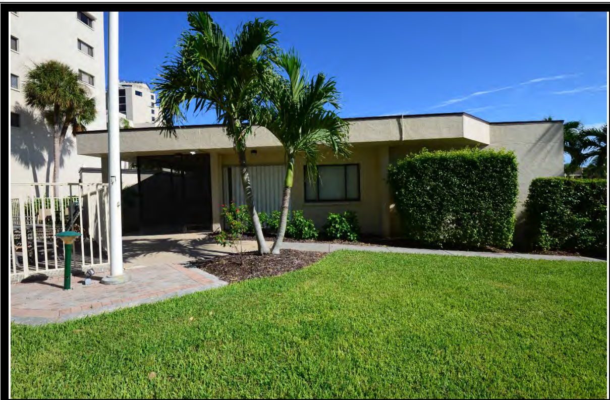
VIEW OF OFFICE/MANAGER'S APARTMENT
