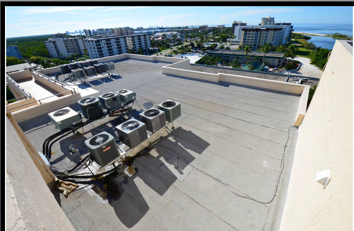
VIEW OF TYPICAL ROOFS
