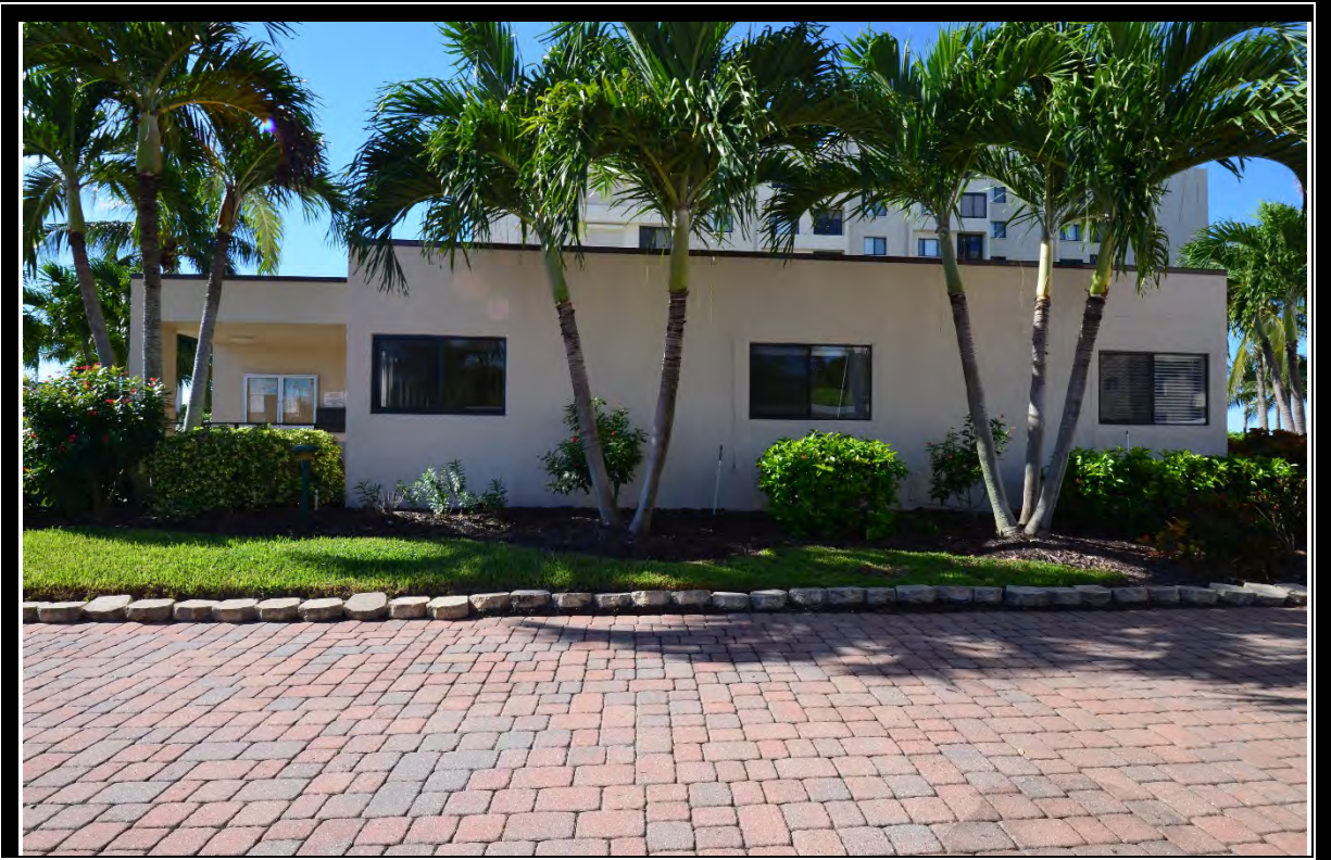
VIEW OF OFFICE/MANAGER'S APARTMENT
