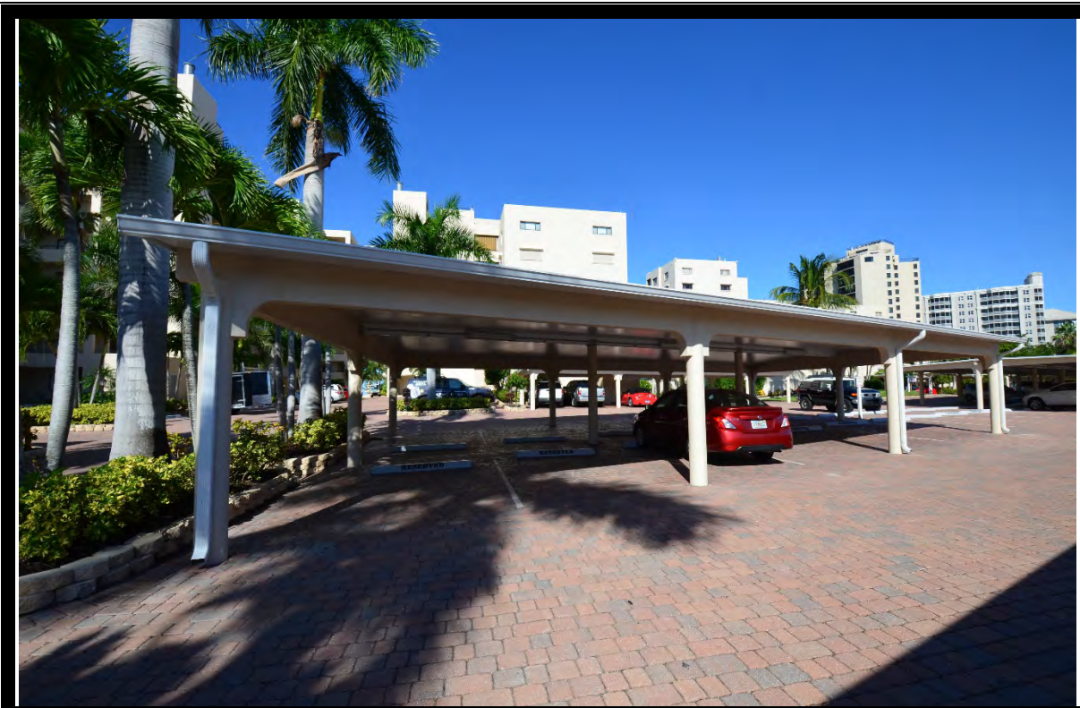
VIEW OF TYPICAL CARPORT STRUCTURES
