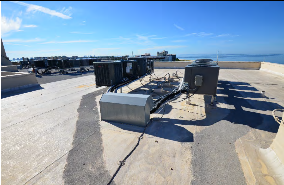
VIEW OF TYPICAL ROOFS
