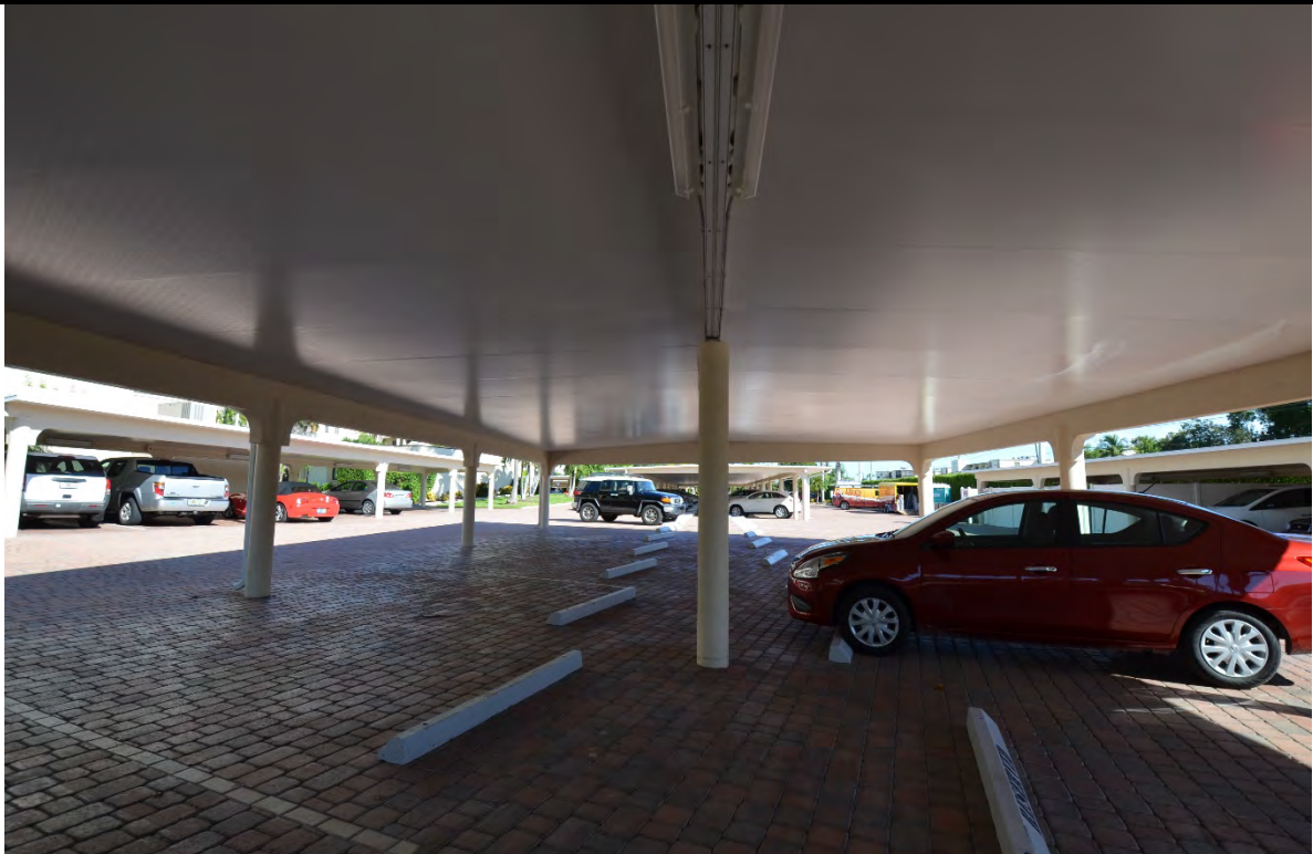
VIEW OF TYPICAL CARPORT STRUCTURES
