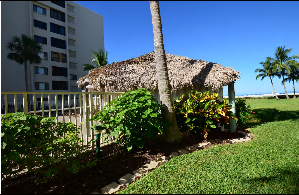
VIEW OF POOL EQUIPMENT CABANA
