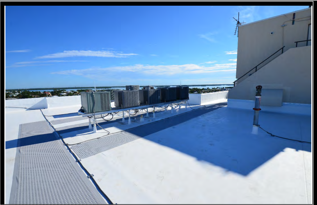
VIEW OF TYPICAL ROOFS
