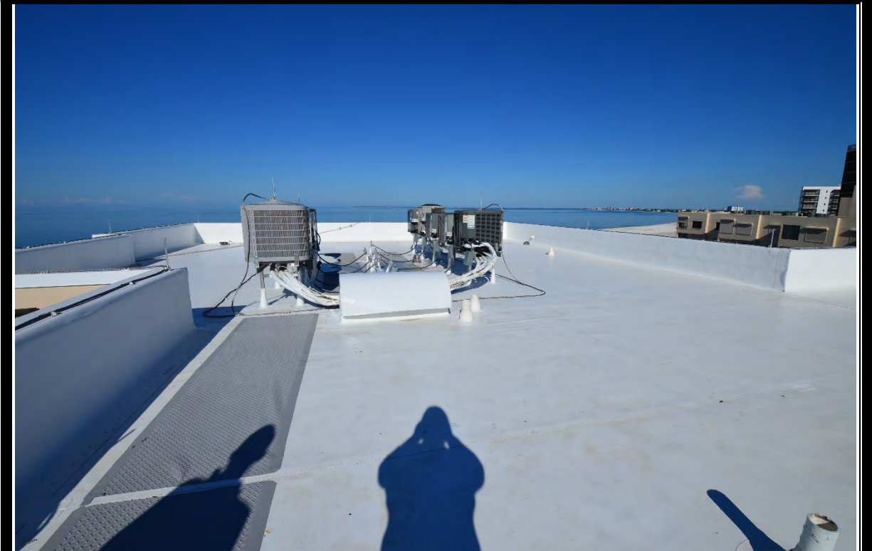
VIEW OF TYPICAL ROOFS
