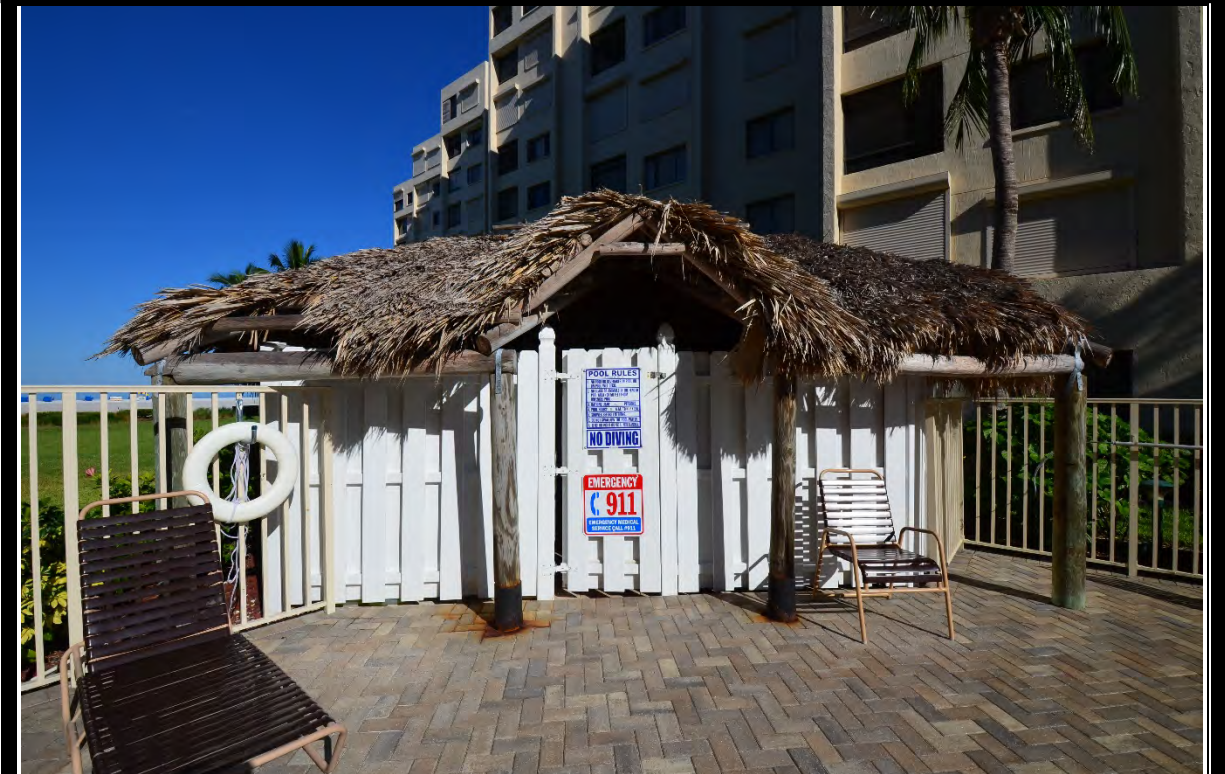
VIEW OF POOL EQUIPMENT CABANA
