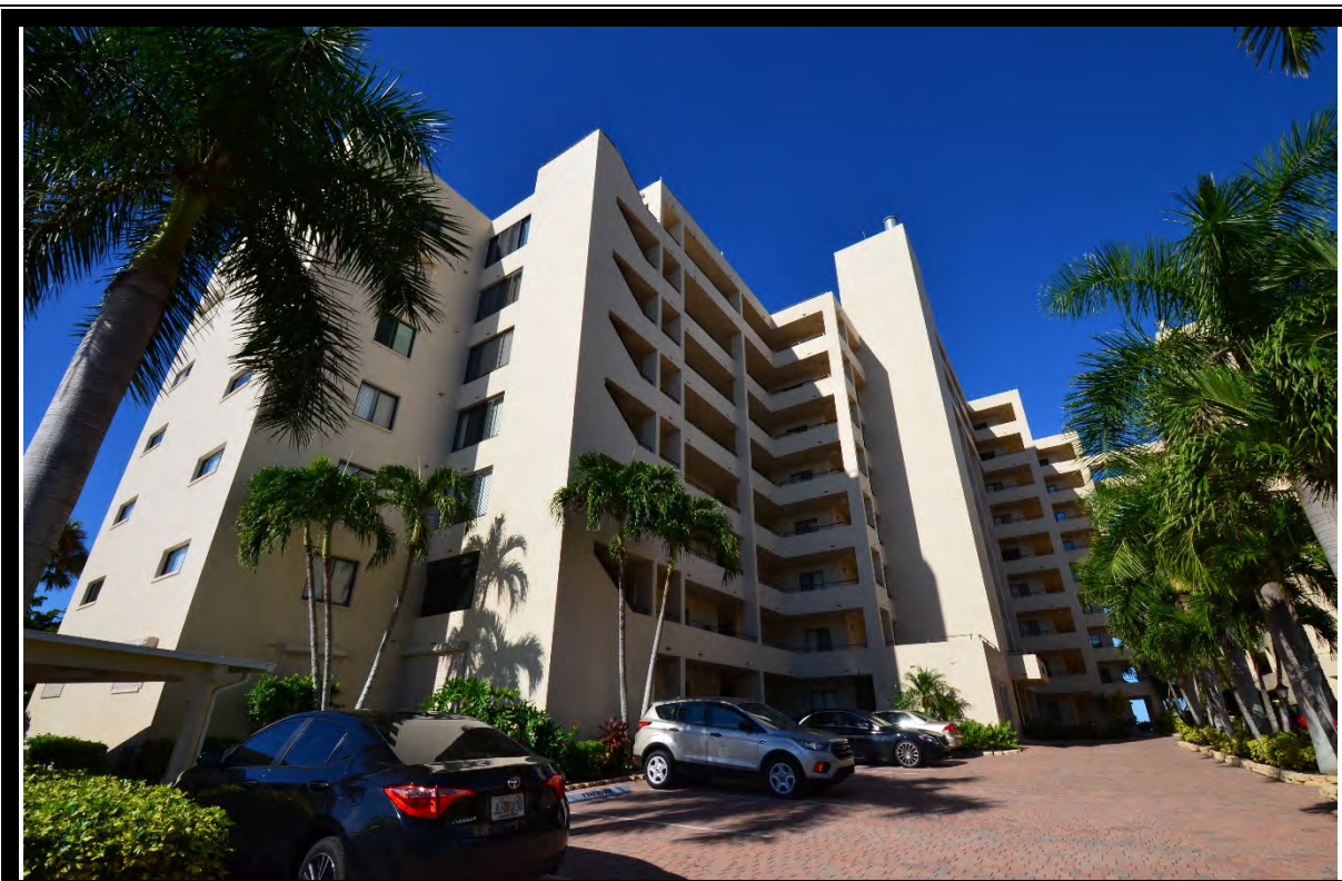
EXTERIOR VIEW OF 6672 ESTERO BOULEVARD 50 UNIT RESIDENTIAL BUILDING
