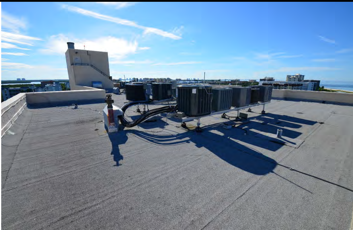
VIEW OF TYPICAL ROOFS
