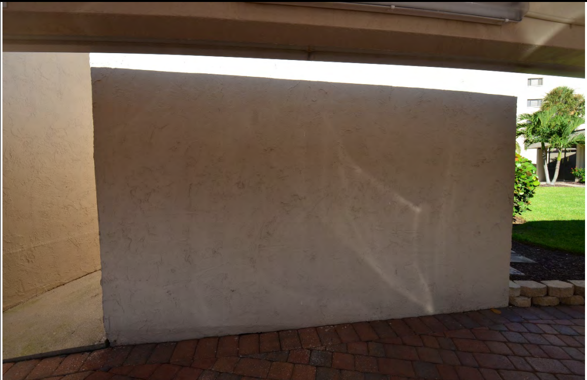
VIEW OF GENERATOR BUILDING
