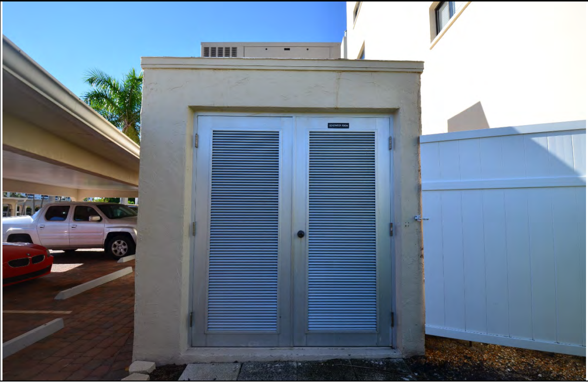
VIEW OF GENERATOR BUILDING
