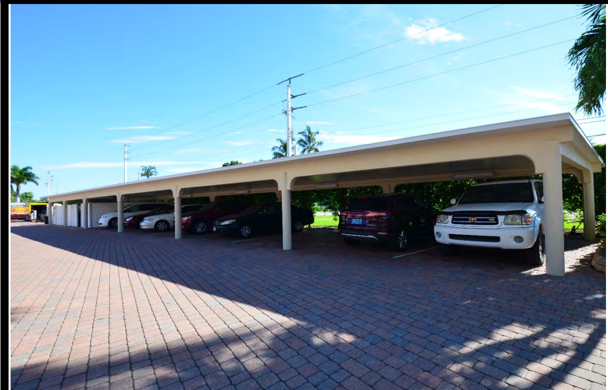
VIEW OF TYPICAL CARPORT STRUCTURES
