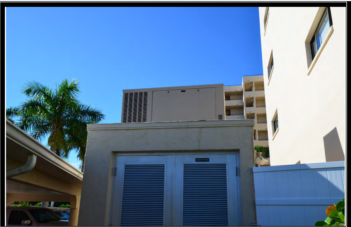
VIEW OF GENERATOR BUILDING
