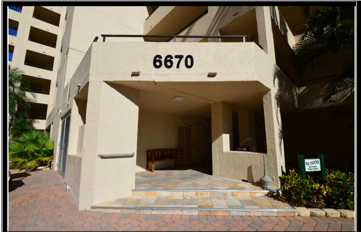
EXTERIOR VIEW OF 6670 ESTERO BOULEVARD 38 UNIT RESIDENTIAL BUILDING
