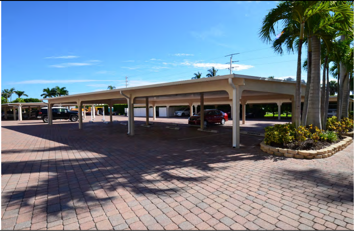
VIEW OF TYPICAL CARPORT STRUCTURES
