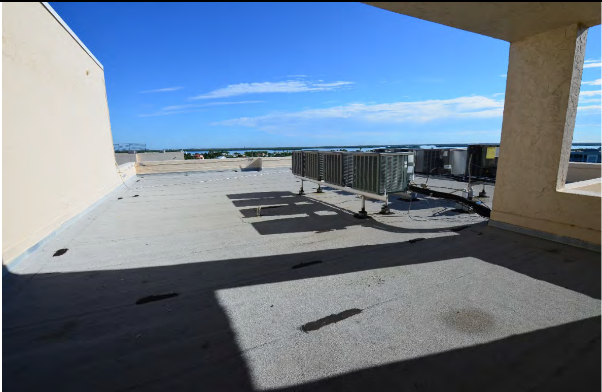
VIEW OF TYPICAL ROOFS
