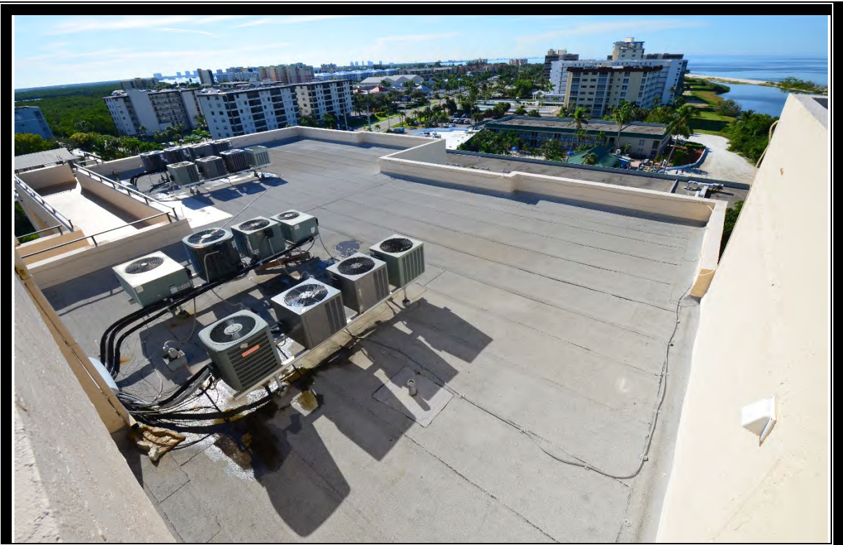
VIEW OF TYPICAL ROOFS
