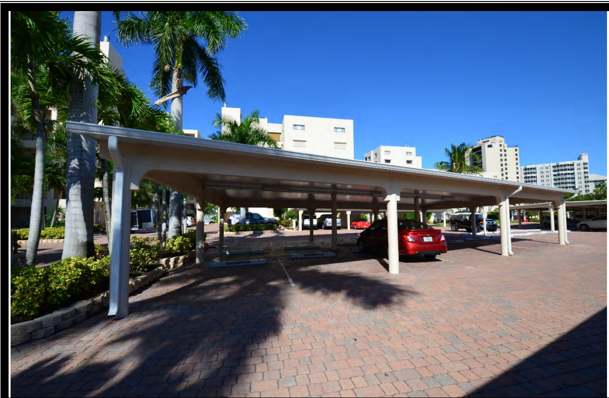
VIEW OF TYPICAL CARPORT STRUCTURES
