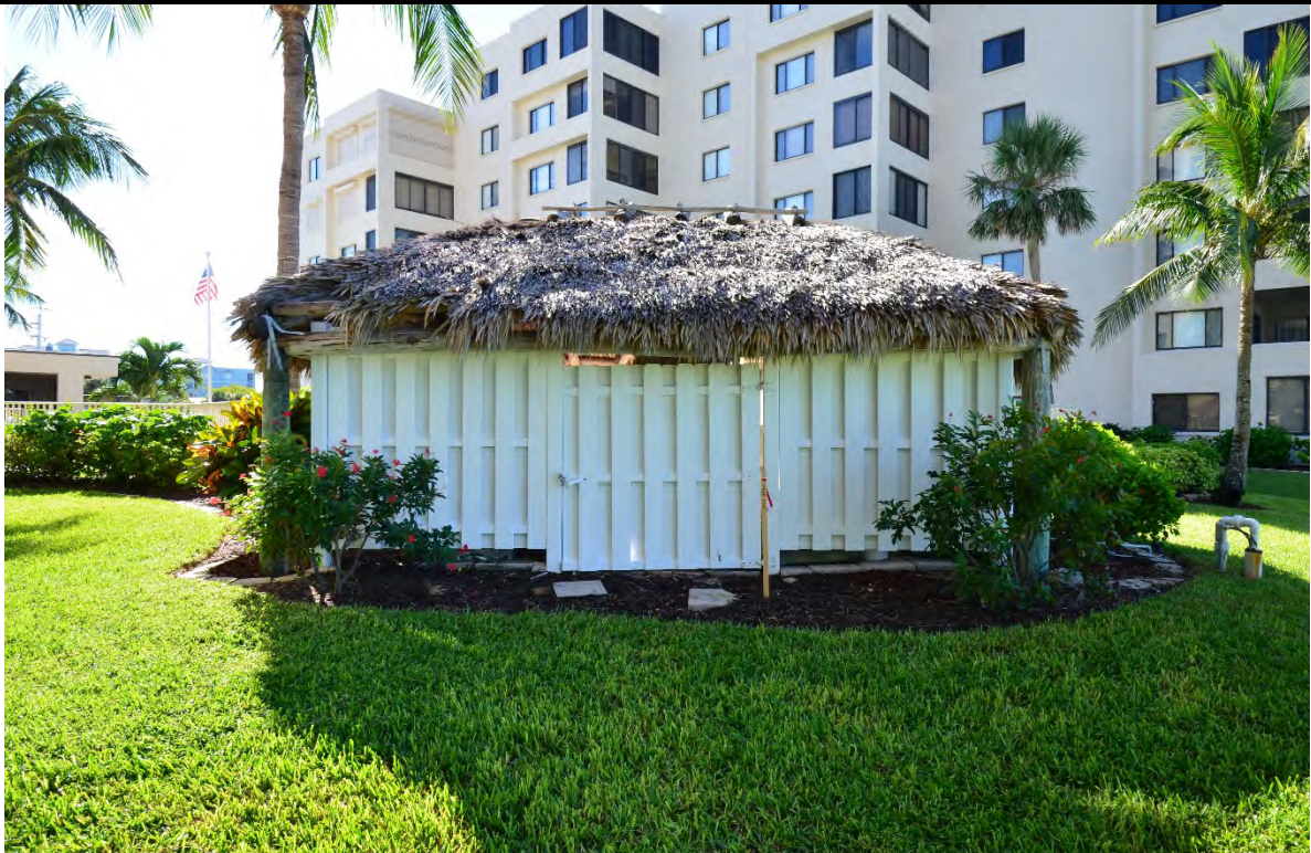
VIEW OF POOL EQUIPMENT CABANA
