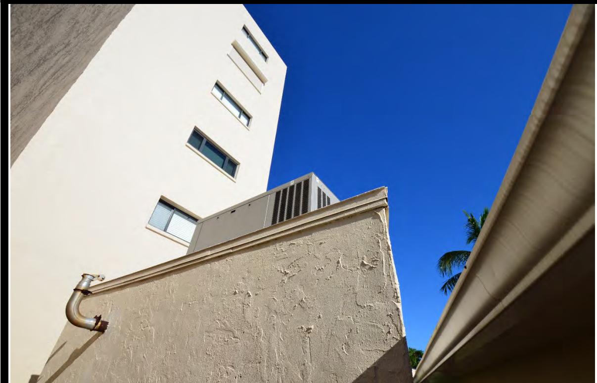
VIEW OF GENERATOR BUILDING
