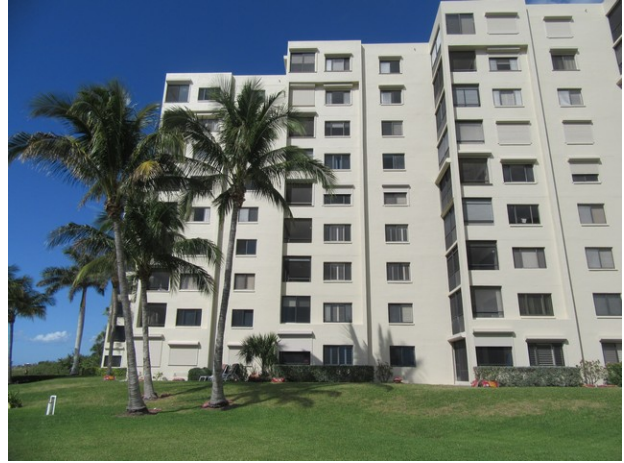
Building exterior overview
