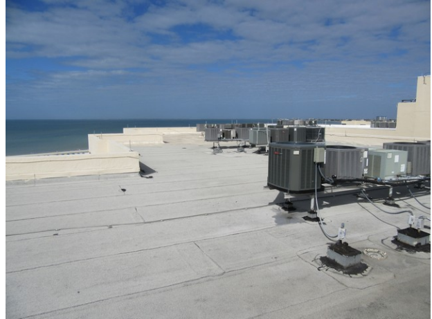
Modified bitumen roof
