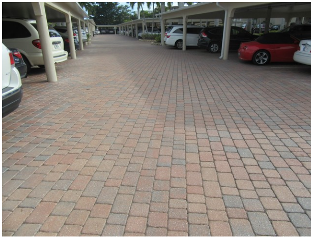
Masonry paver driveway and parking areas
