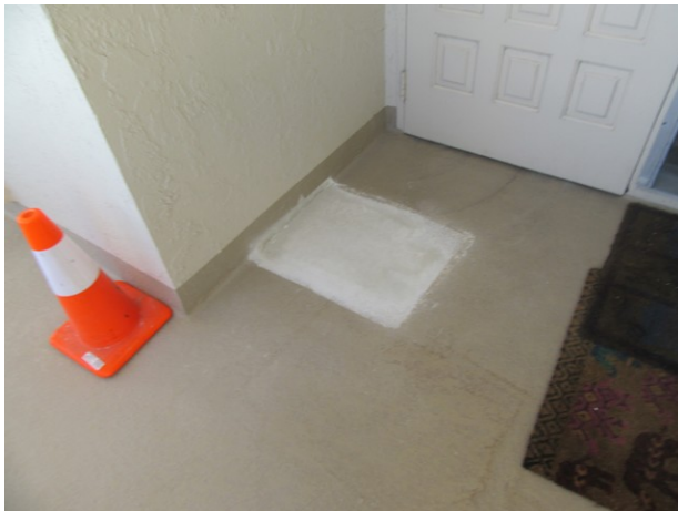
Concrete repair at Unit A 810 entrance
