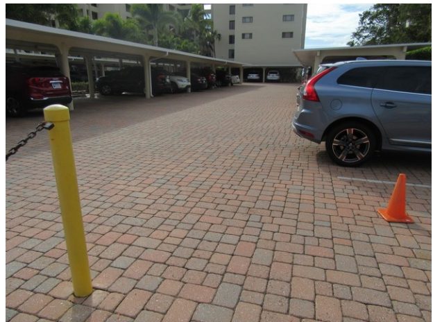
Masonry paver driveway and parking areas
