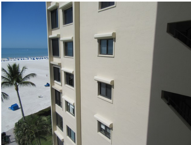
Exterior stucco walls
