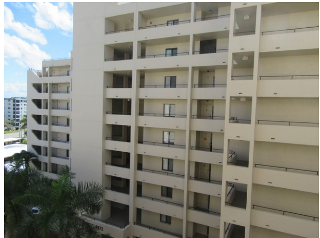
Building exterior overview
