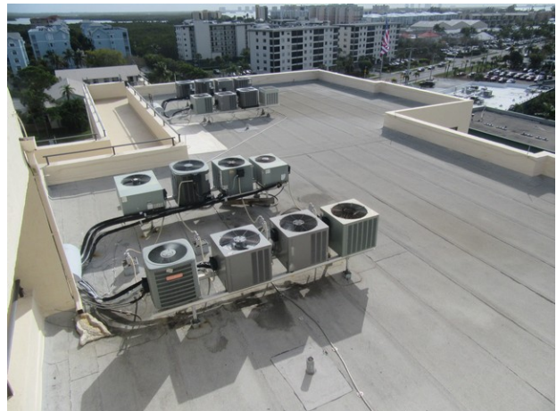
Modified bitumen roof
