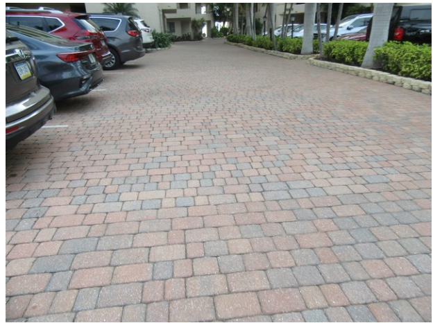
Masonry paver driveway and parking areas
