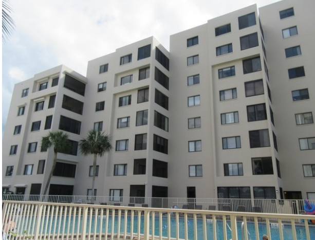
Building exterior overview
