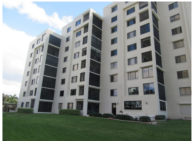
Building exterior overview
