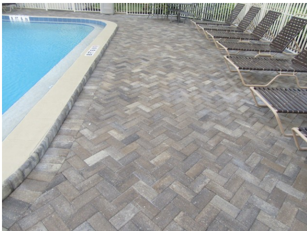
Masonry paver pool deck
