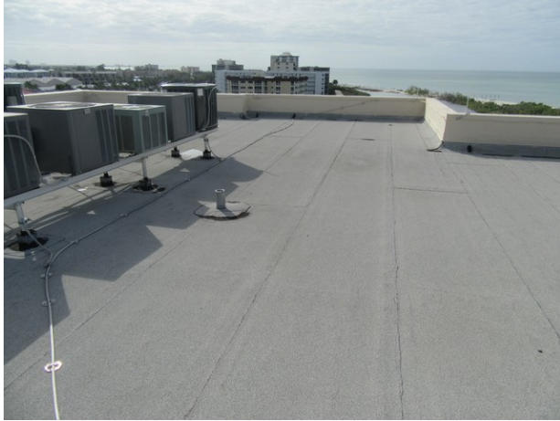
Modified bitumen roof
