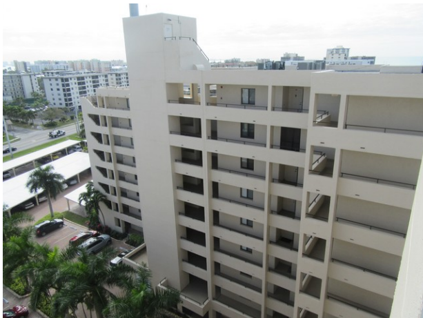
Building exterior overview
