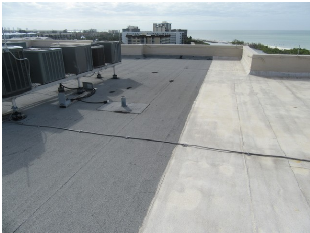
Modified bitumen roof (roof stack 6 with coating on right)
