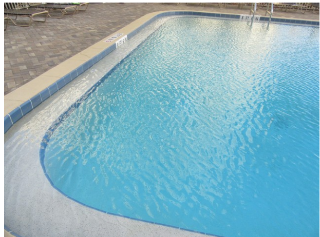
Pool plaster finish
