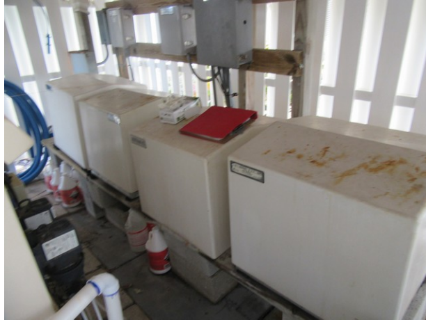
Geothermal heaters
