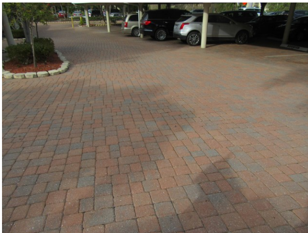
Masonry paver driveway and parking areas
