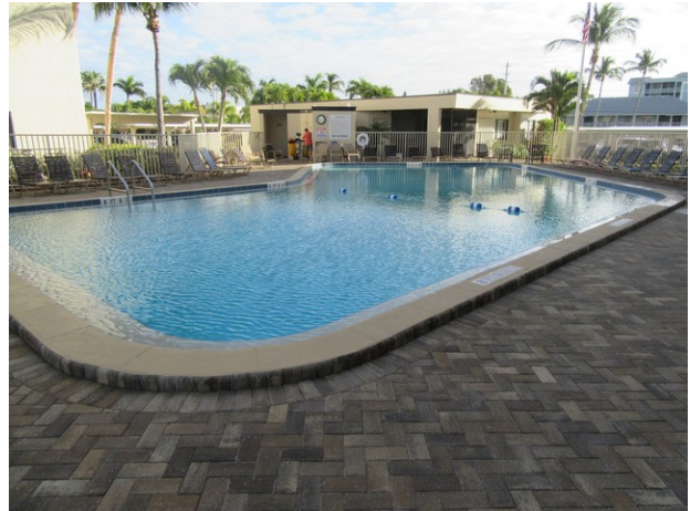
Pool area overview
