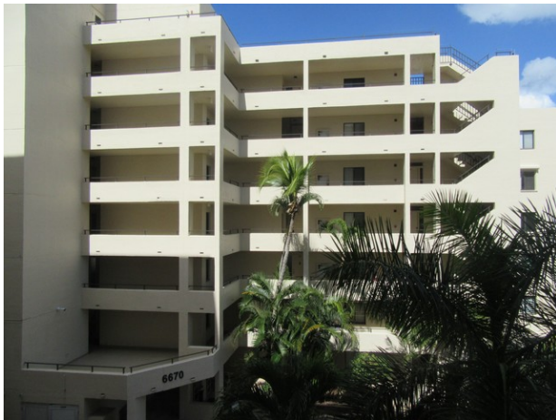
Building exterior overview
