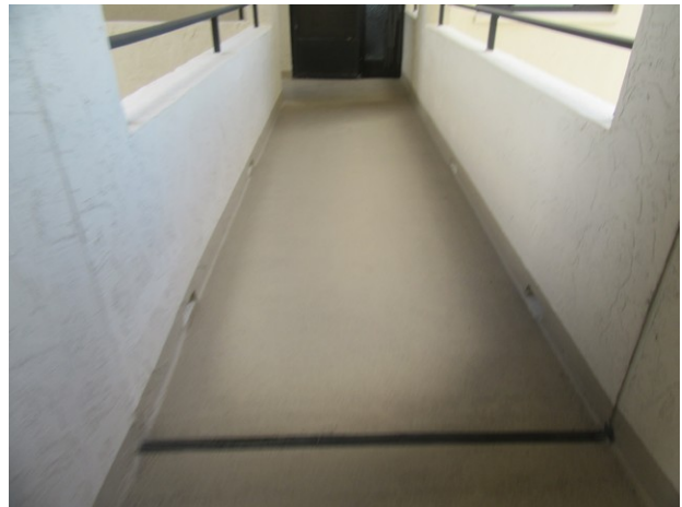
Breezeway with waterproof coating
