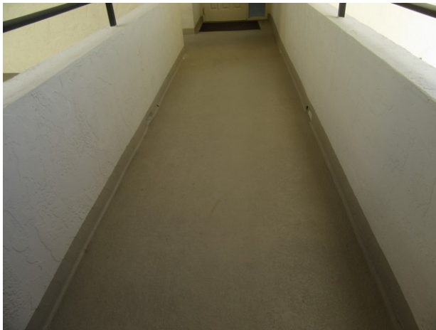
Breezeway with waterproof coating
