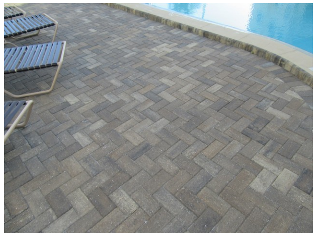
Masonry paver pool deck
